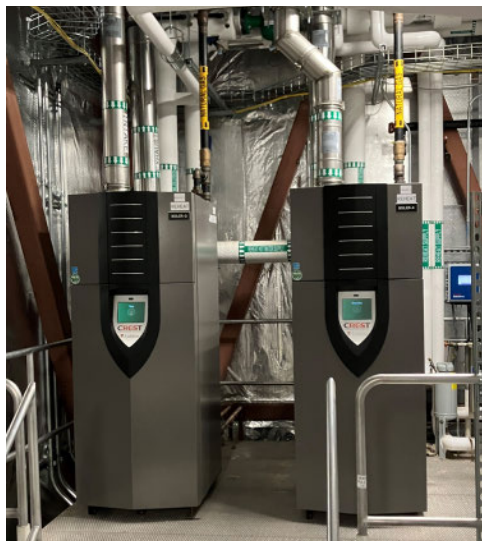
The reheat boilers in Bldg. T30
